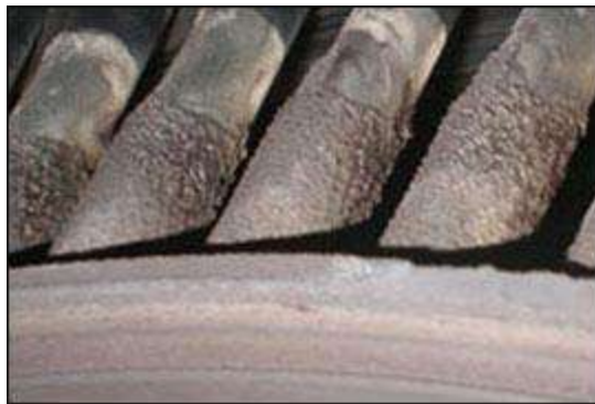
Figure 1. Amorphous silica deposits on steam turbines. Reproduced with permission from https://tofanhakim.wordpress.com .
