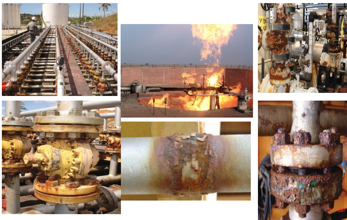
Figure 1. Examples of flanges, valves and welded joint corrosion.
