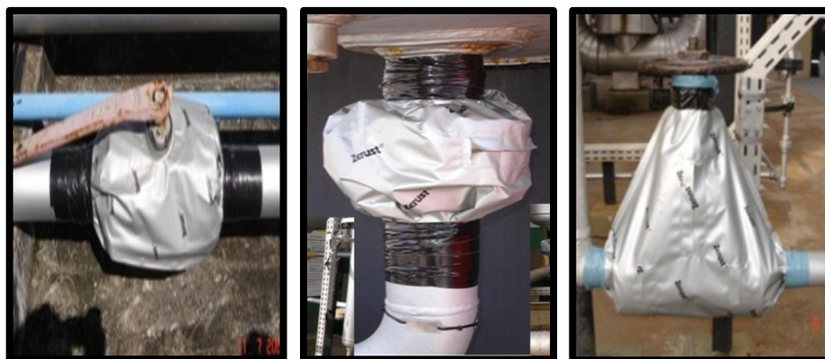
Figure 4. Various configurations of FPS cover installation.
