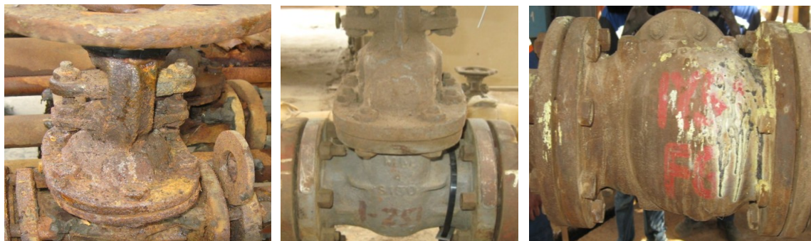
Figure 6. Typical corrosion condition of the flanges/valves.
